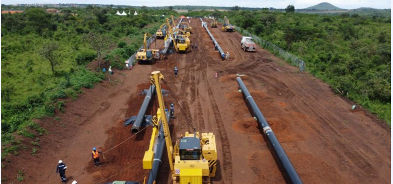
Picture showing EACOP pipes being aligned. Photo credit Deep Earth
